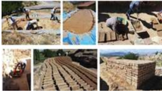
Figure 4. Production line of 2019 the mud bricks of Zeyve Höyük (© Porsuk – Zeyve Höyük archaeological mission)
