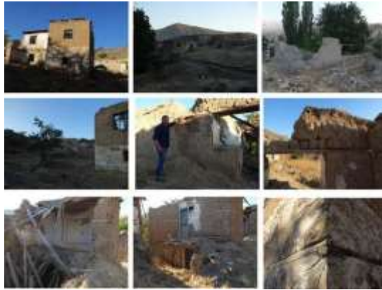
Figure 5. Houses and constructive details of Eski Porsuk village (© CRAterre_C. Sadozai)
