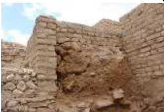
Figure 6: Encapsulation of the original Hittite mud bricks (© Porsuk – Zeyve Höyük archaeological mission)
